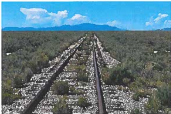
Figure 4 - North End - Photograph at MP 22
