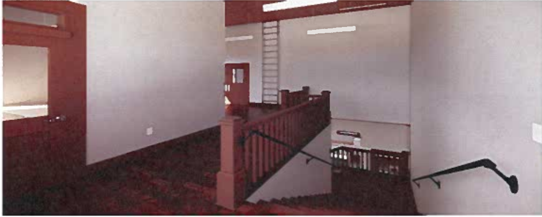
Historic Stair - View From Top of Stair April 25, 2024
