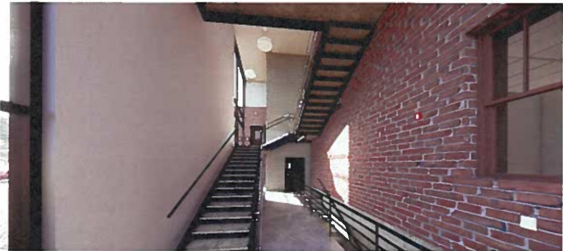
Stair Tower - View From First Floor Landing April 25, 2024
